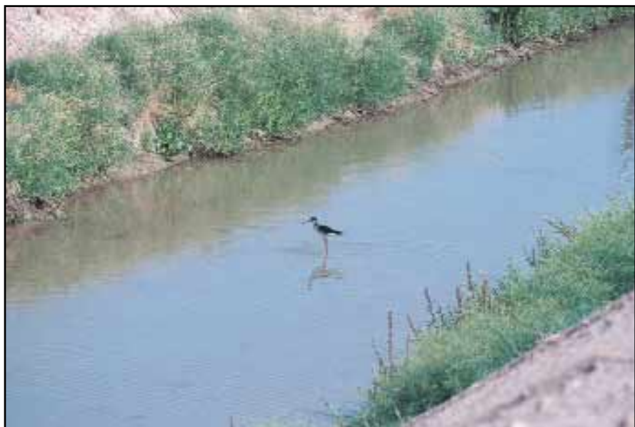
Fig. 11. Stilt in drainage canal.
