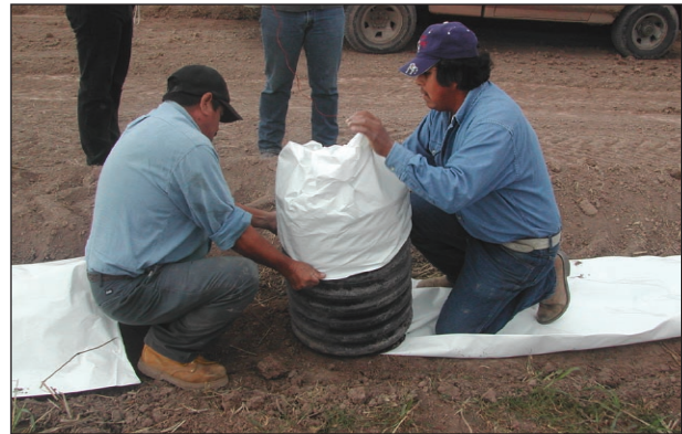
Figure 5a. Connecting two rolls of poly-pipe.
