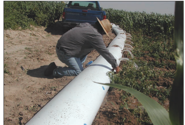
Figure 8a. Inserting plugs in poly-pipe.
