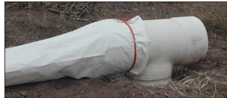
Figure 4b. Using rubber straps to connect the poly-pipe to the supplying pipe.
